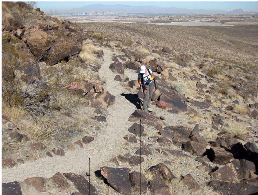
COMPACTED NATURAL SOIL TRAIL TREAD
